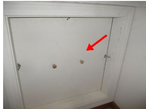
Insulate access panel to attic
