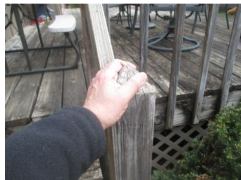
Loose handrail
