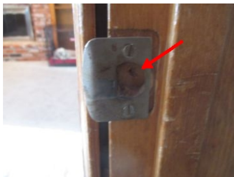
Realign strike plate for doors that won't latch
