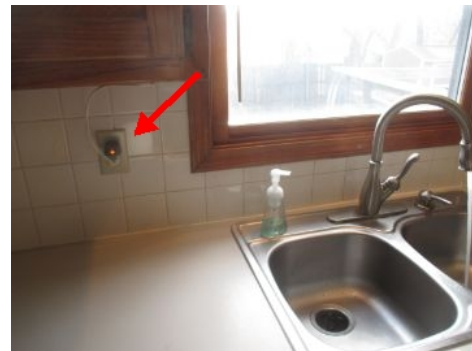
Install GFIs in kitchen on both sides of sink
