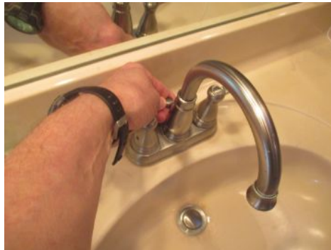
Inoperative lift rod in master bath
